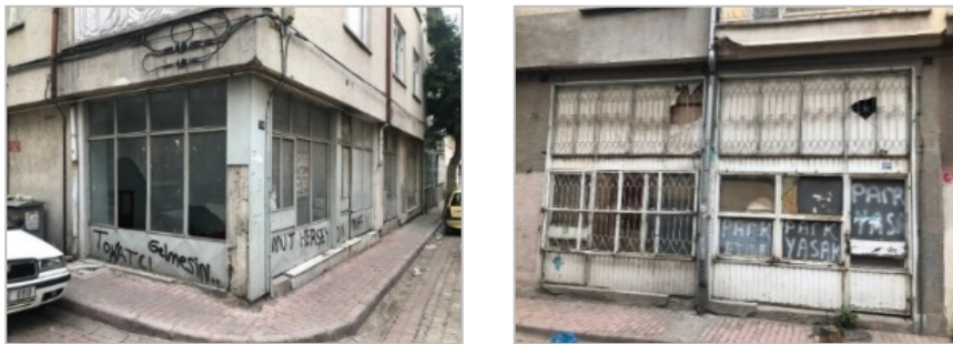
Figure 9. Vandalism acts in the area
