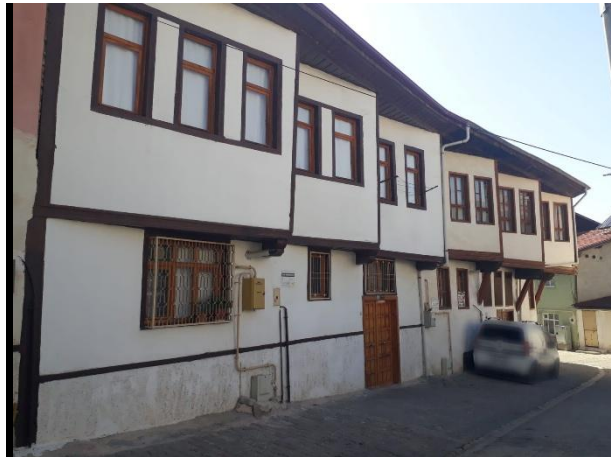
Figure 2. An example showing the differentiation of ground floor and upper floor facade layouts due to privacy in traditional houses, Tokat
