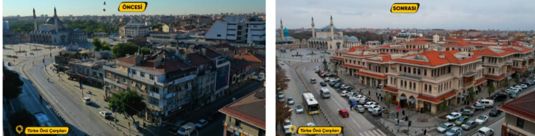
Figure 9. Tırbeönü Bazaar renovation project- before and after
