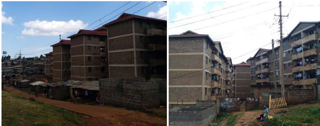
Figure 10. The Newly Built Houses in Soweto, Kibera.
