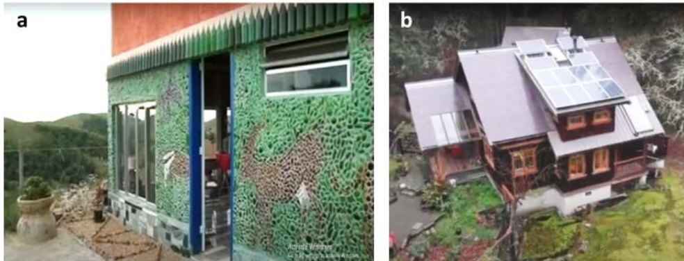
Figure 1. Buildings A & B
