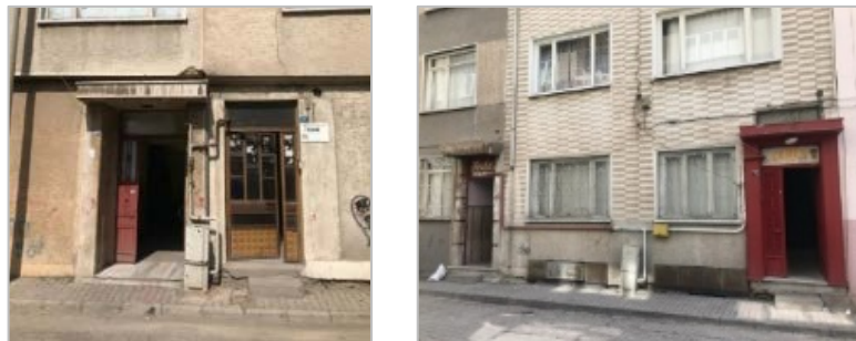
Figure 6. Entrance door and window examples
